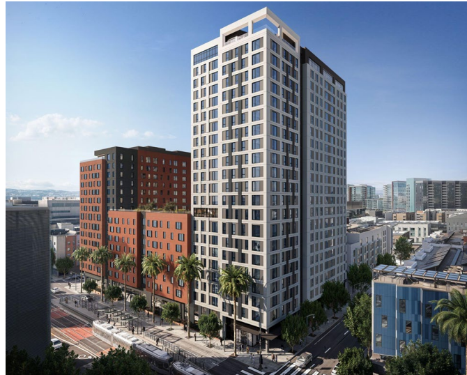
Mission Bay South Block 4E Phase II
