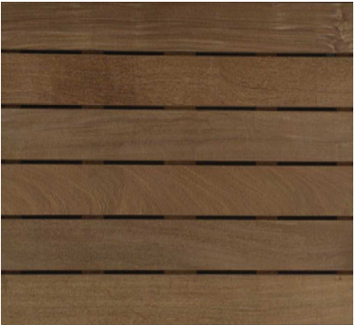
IPE DECKING ON FRONT BALCONIES, BACK ROOFTOP DECK, AND PERGOLA ROOF
