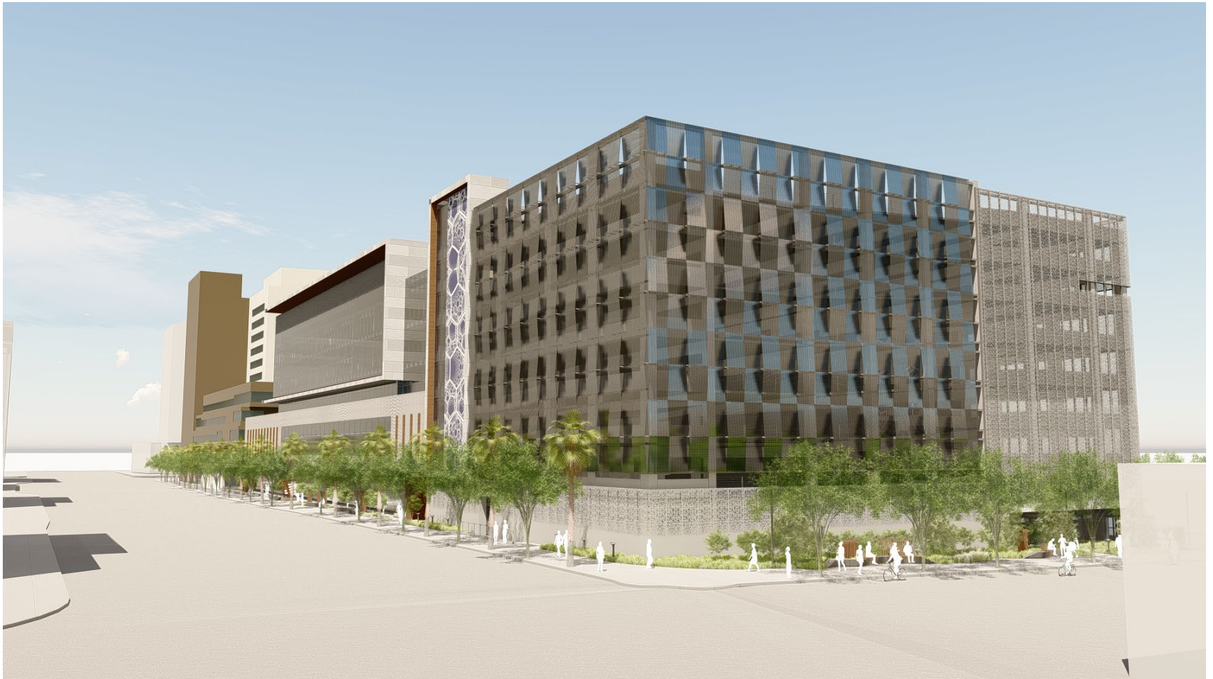
Southwest Corner View from Third Street – Gateway Corner
