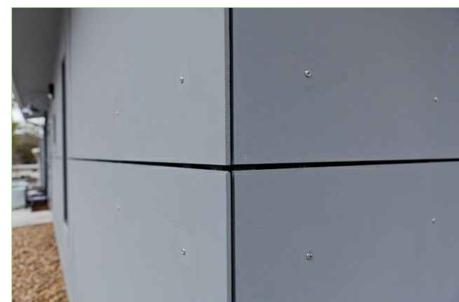
RAIN SCREEN (CORNER DETAIL)
