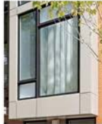
BRONZE ANODIZED CUSTOM ALUMINUM WINDOWS BY "ALLWEATHER SERIES 5000" OR EQ.
