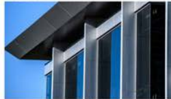
ALUMINUM RAINSCREEN SYSTEM BY ALUMAWALL 1800 SERIES
