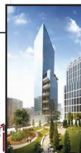
Block 5 250 Howard Street Park Tower
