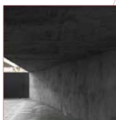
Grand Entry Canopy: Precast Concrete
