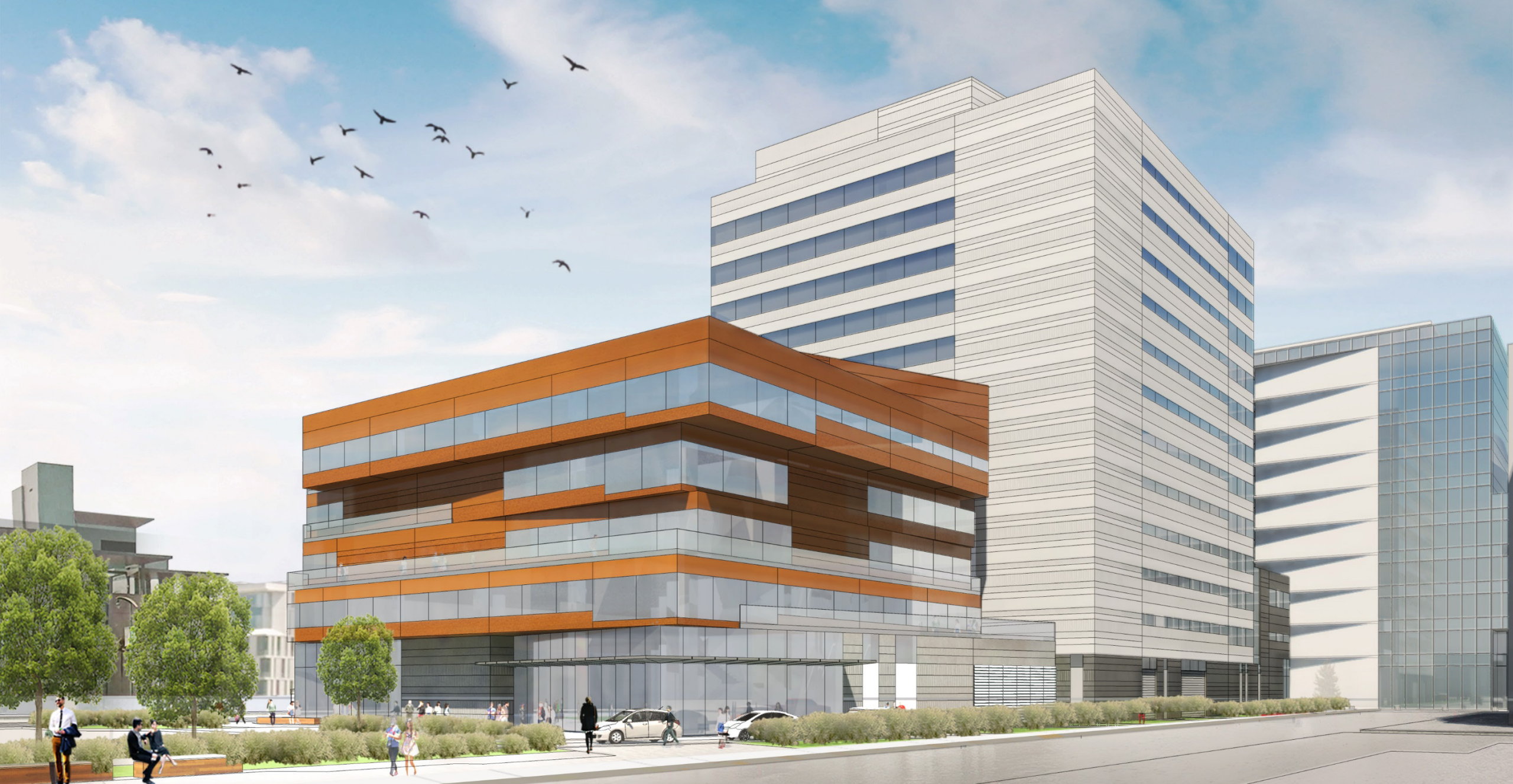
View from Illinois Street Looking Northwest
