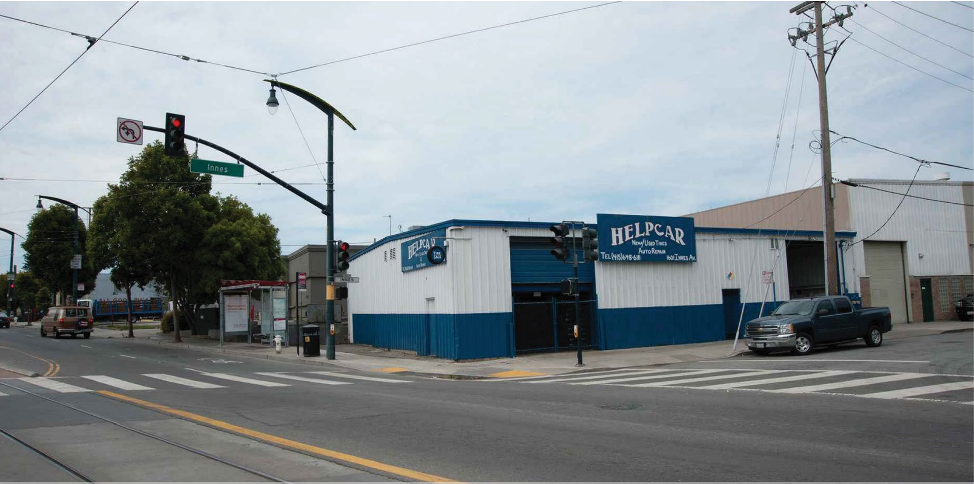
View from Corner of Third Street & Innes Ave
