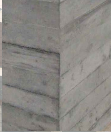
BOARD FORM CONCRETE
