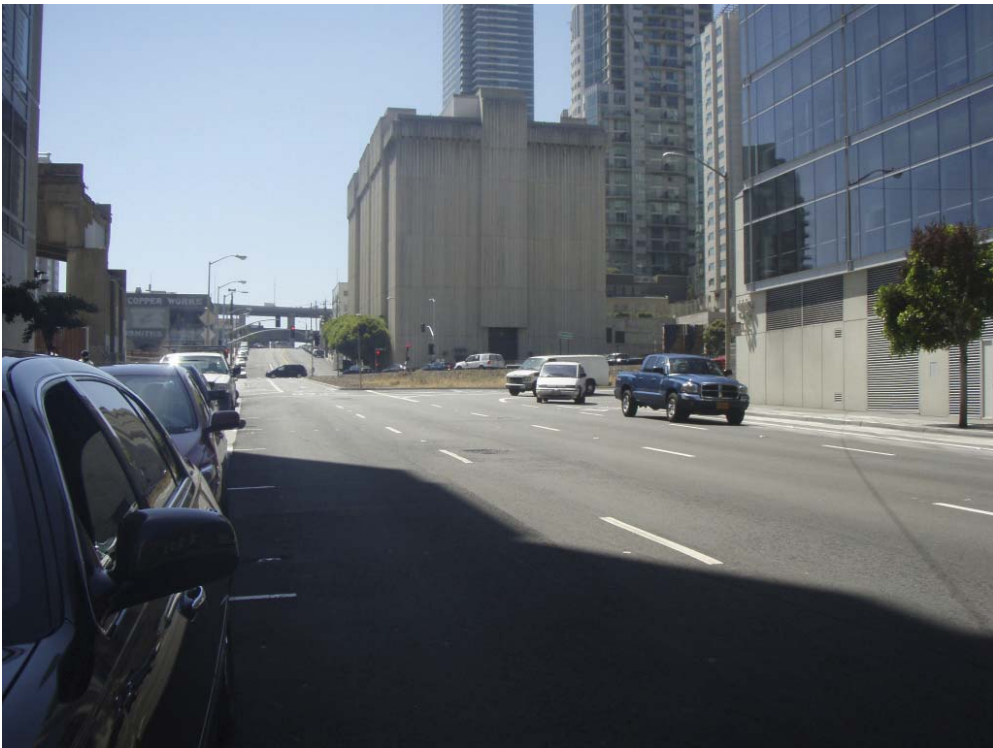
Looking west at offramp from the Folsom Street/Fremont Street intersection
