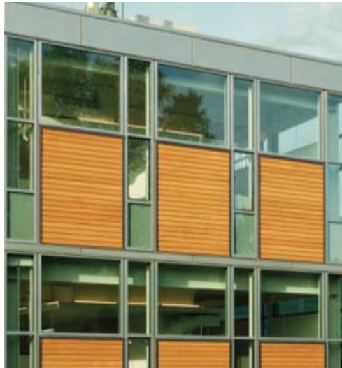
Coated metal window framing to match panels; clear low-e glass
