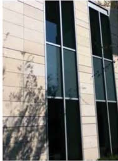
EXAMPLES: OPEN JOINT PANEL SYSTEM WITH STOREFRONT
