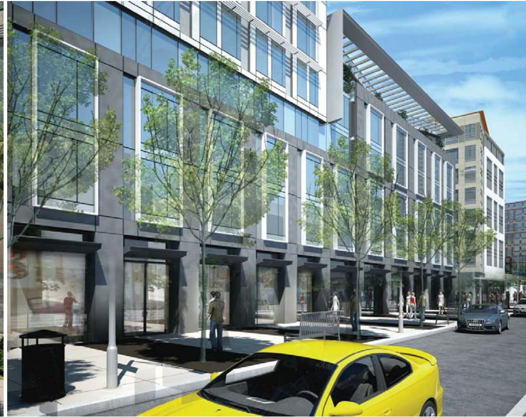
FOLSOM STREET LOOKING NORTH
