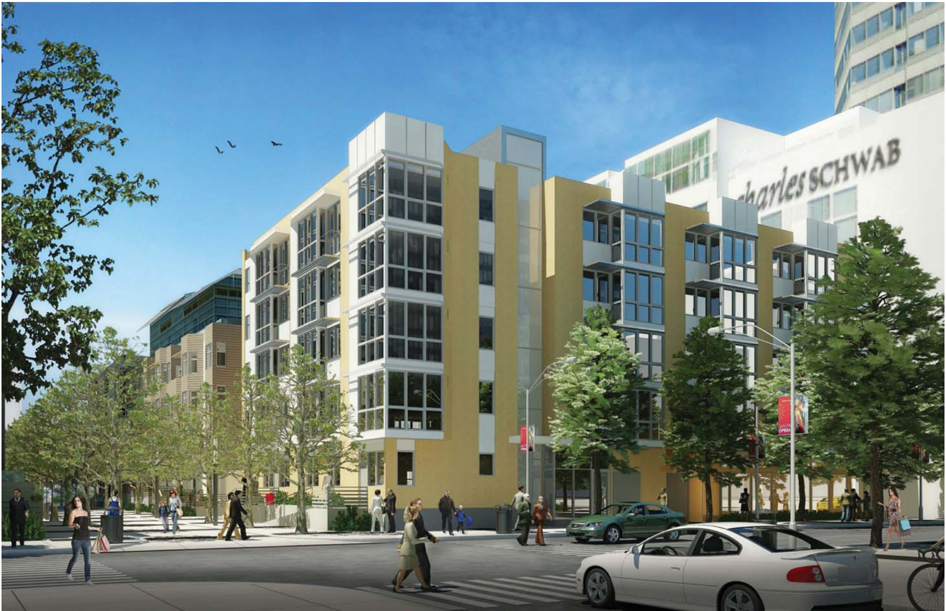
BUILDING 7B FROM BEALE STREET
