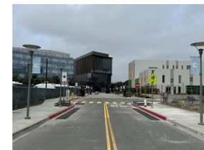
Roadway striping and finished approaches
