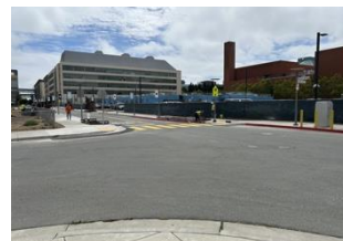
New crosswalk and accessible corner details
