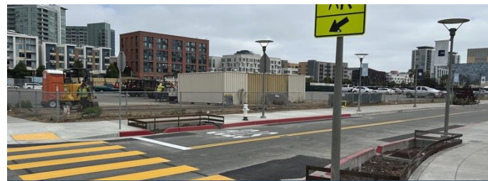
Completed intersection • pedestrian crossing + curb improvements
