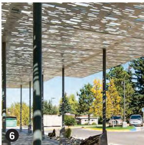
6 TRELLIS WITH CUSTOM LASER CUT PATTERN CANOPY
